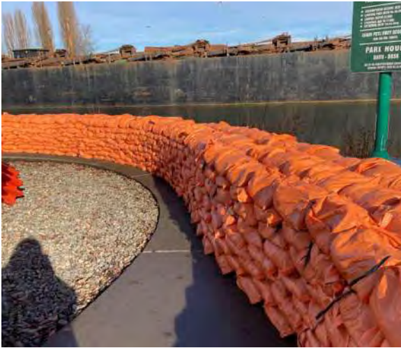
Emergency preparedness efforts including temporary sandbag walls to protect from river flooding (SPU & King County)
