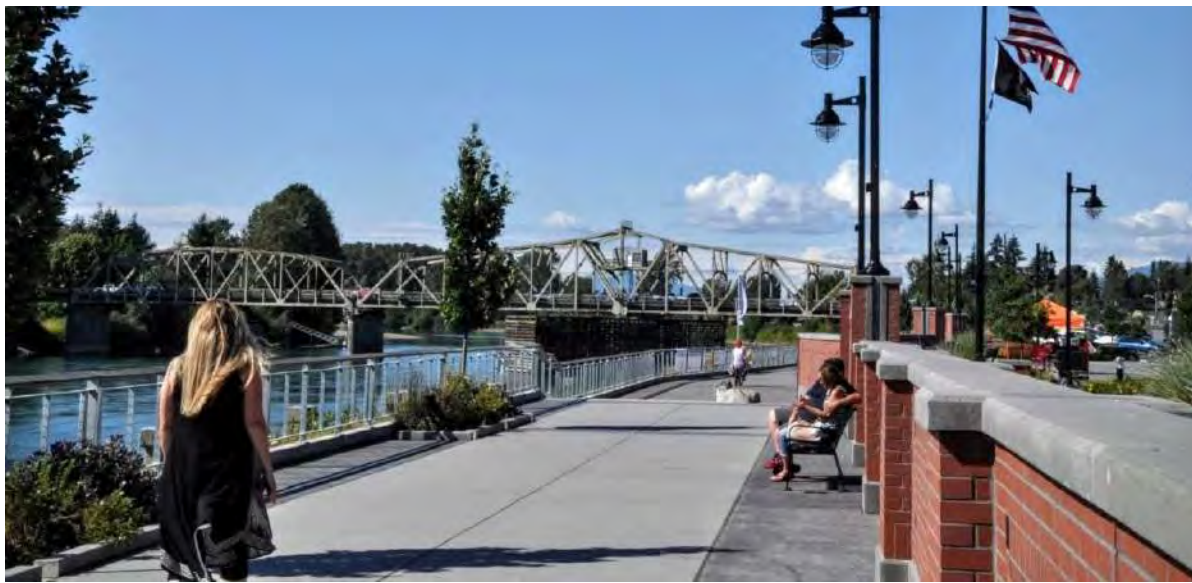
Riverwalk levee that includes a flood wall on top, providing additional protection height. Mt. Vernon, WA
