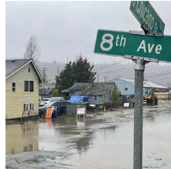
Existing homes within the industrial zone are particularly exposed to high-tide flooding today.
