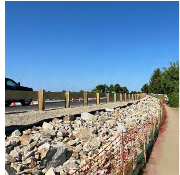
Example: Peirce Island Road, Portsmouth, NH
