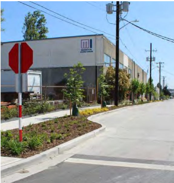
Drainage and Roadway Improvements (SPU/SDOT)
