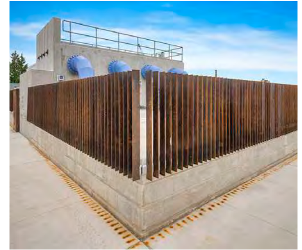
South Park Pump Station (SPU)
