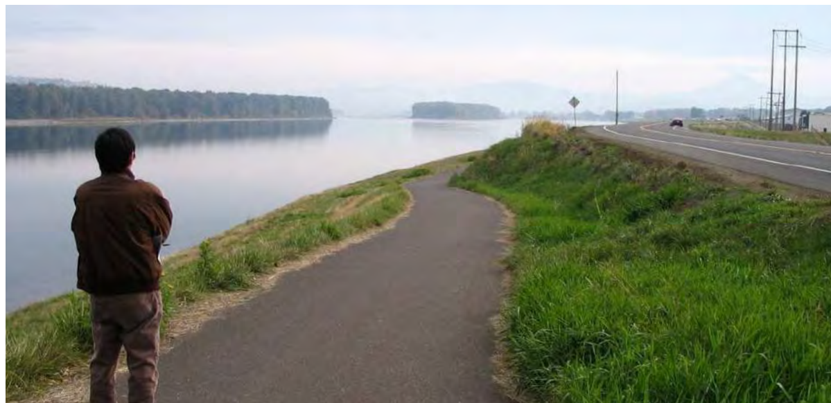
Marine Drive raised road along Columbia River, Portland, OR
