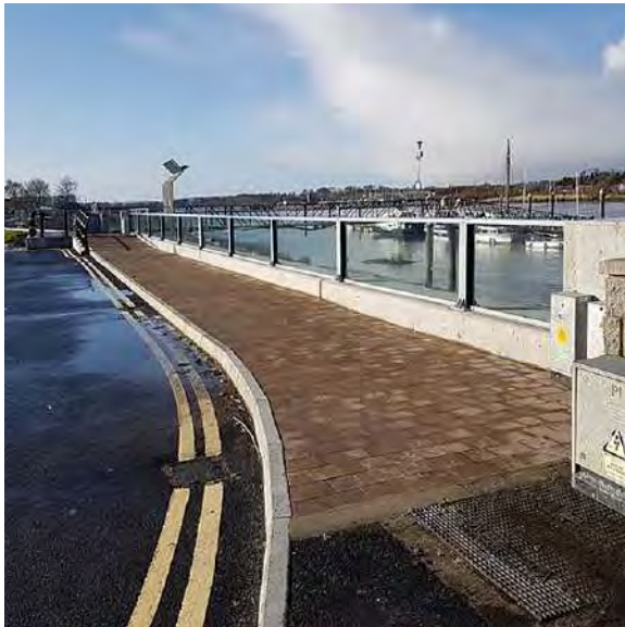
Flood walls can add height to a raised road or levee
